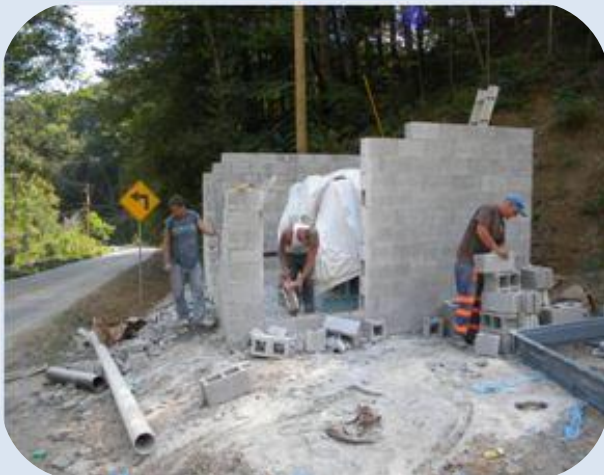
Workers (left) construct one of the four pump stations to force water up the mountain to the water tank being built at the top of Black Mountain (right). Photos by David Messer and Ryan Wilson, DOW field inspectors at the London Regional Office.
