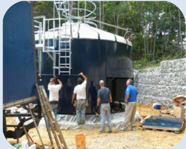
Workers (left) construct one of the four pump stations to force water up the mountain to the water tank being built at the top of Black Mountain (right). Photos by David Messer and Ryan Wilson, DOW field inspectors at the London Regional Office.
