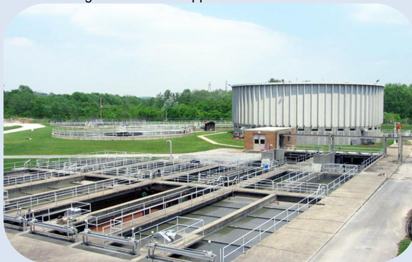
Photo courtesy of Gresham, Smith and Partners
