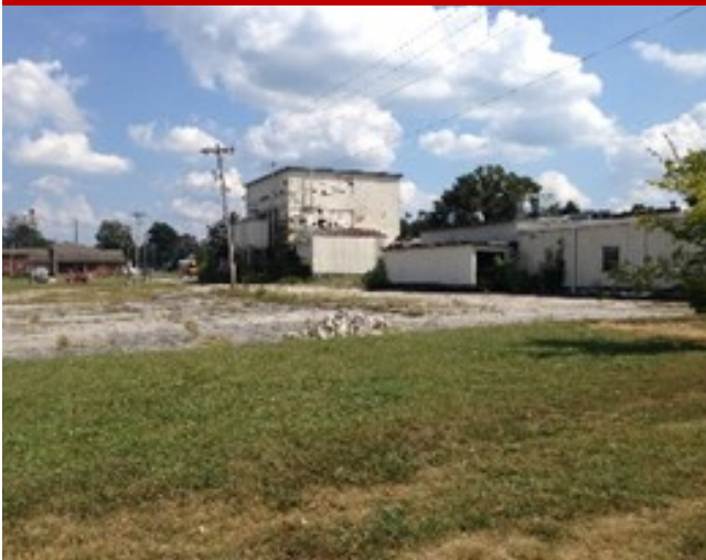
The Parker Seal Rubber Plant in Berea sits awaiting remediation using a US EPA Brownfield Cleanup Grant.
