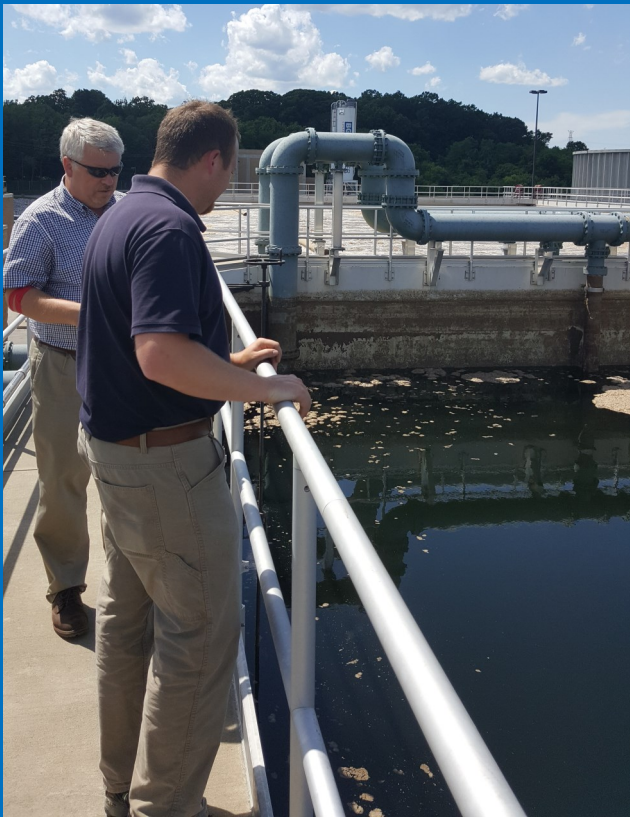
Above: John Durbin and Doug Kimbler at the Bowling Green Wastewater Treatment Plant.
