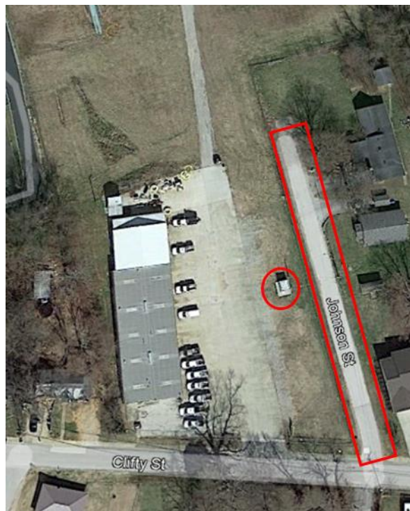
Figure 2: Google Earth image of the Somerset site in relation to Johnson Street. The road dead ends just past two houses located northeast of the site.
