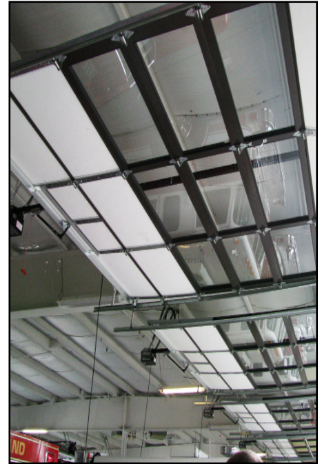
New bay doors with UV glass cost no more than repairing the old ones.
