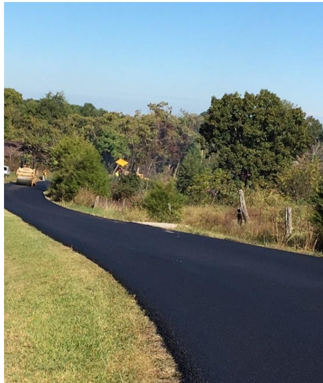
Photo 8: Rubber-modified asphalt project in Green County. Photo by Gary Logsdon
