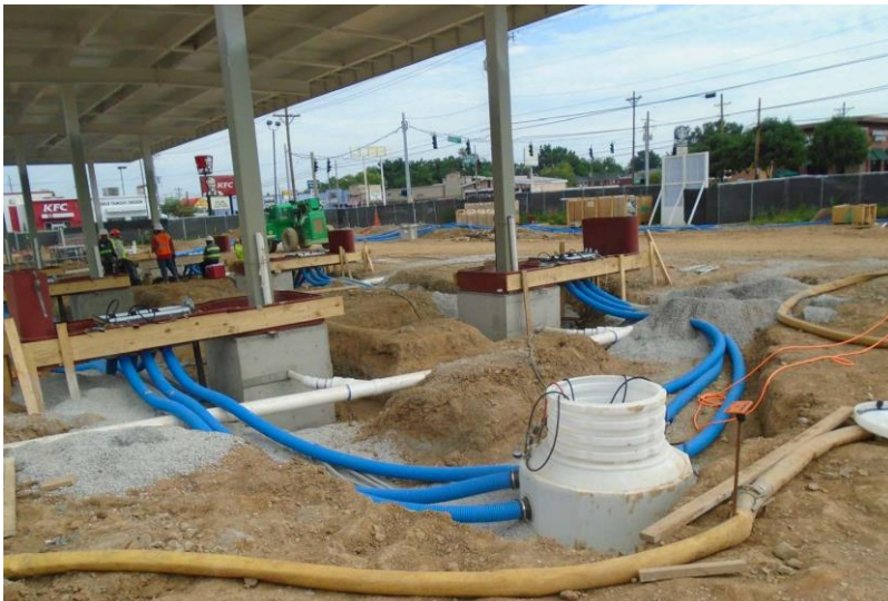
Photo 19: Dispensing area for installment of USTs. Photo by Rob Staley, Field Office Branch
