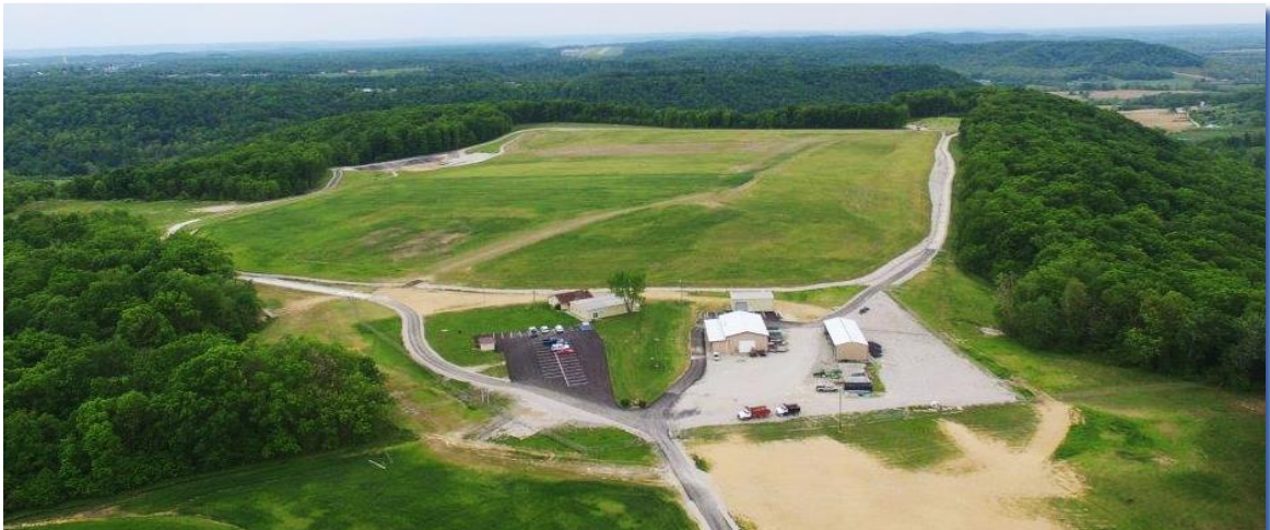
Photo 14: Maxey Flats Project Aerial View of Final Cap Photo by Superfund Branch
