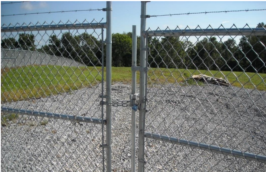
Photo 15: Locked gate, fencing surrounding former production area. Maintenance of cap is one of the primary activities SFB staff perform. At rear of photo from crest to tree line, the slope is steep and subject to erosion. Photo by Superfund Branch
