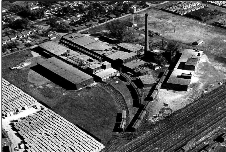
Photo 9: Pre-remediation of Black Leaf Chemical Site
