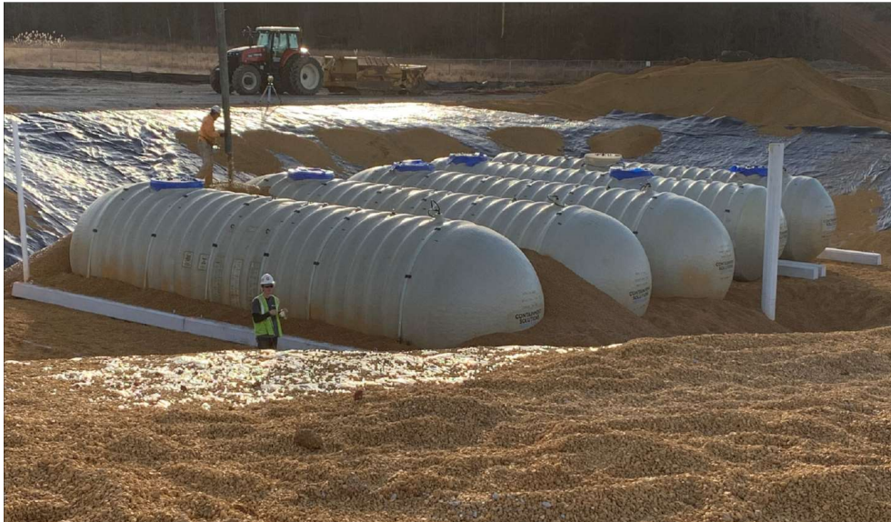
Photo 14: Storage Tank Installation
