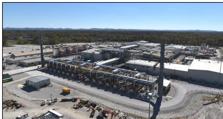
Photo 3 BGCAPP Aerial View
