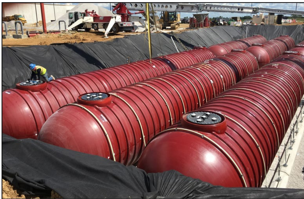
Photo 13 Underground Storage Tank Installation
