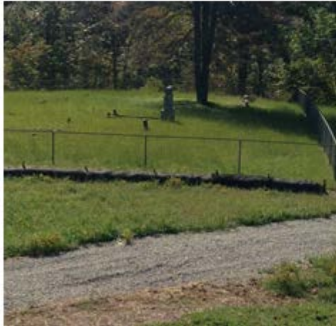
Composite filter sock to prevent sedimentation on cemetery downslope of wellsite
