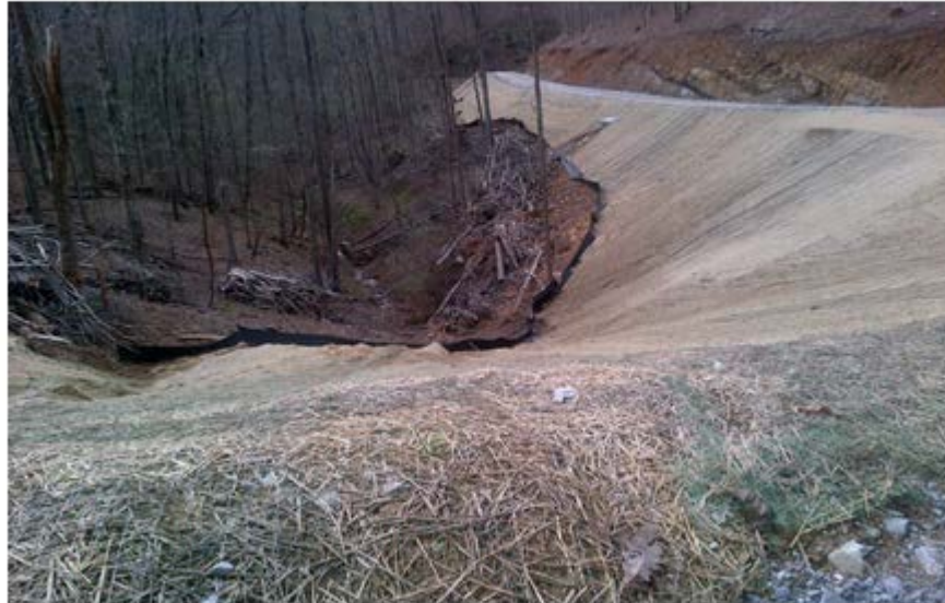
Access road with erosion control matting, silt fence and logs riprap
