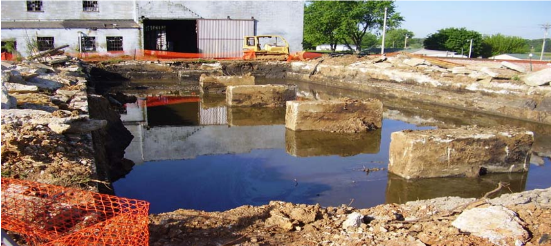
Derby Tank Car Project –prewater removal (before)
