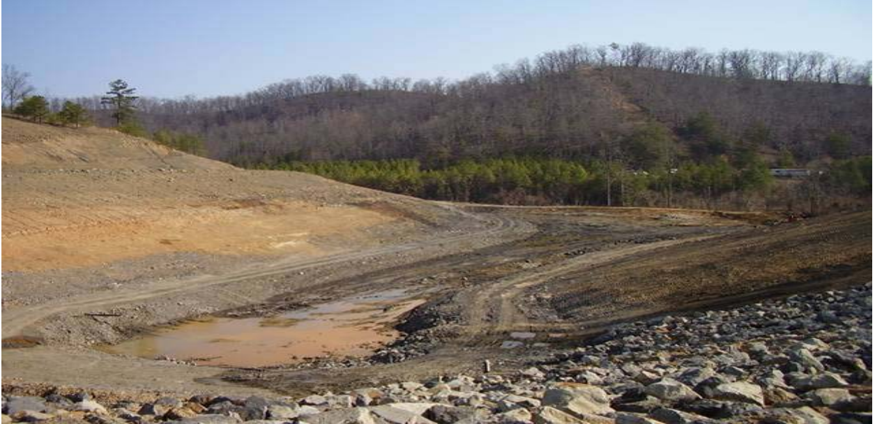
City of Manchester Landfill- Constructed Wetland in Progress
