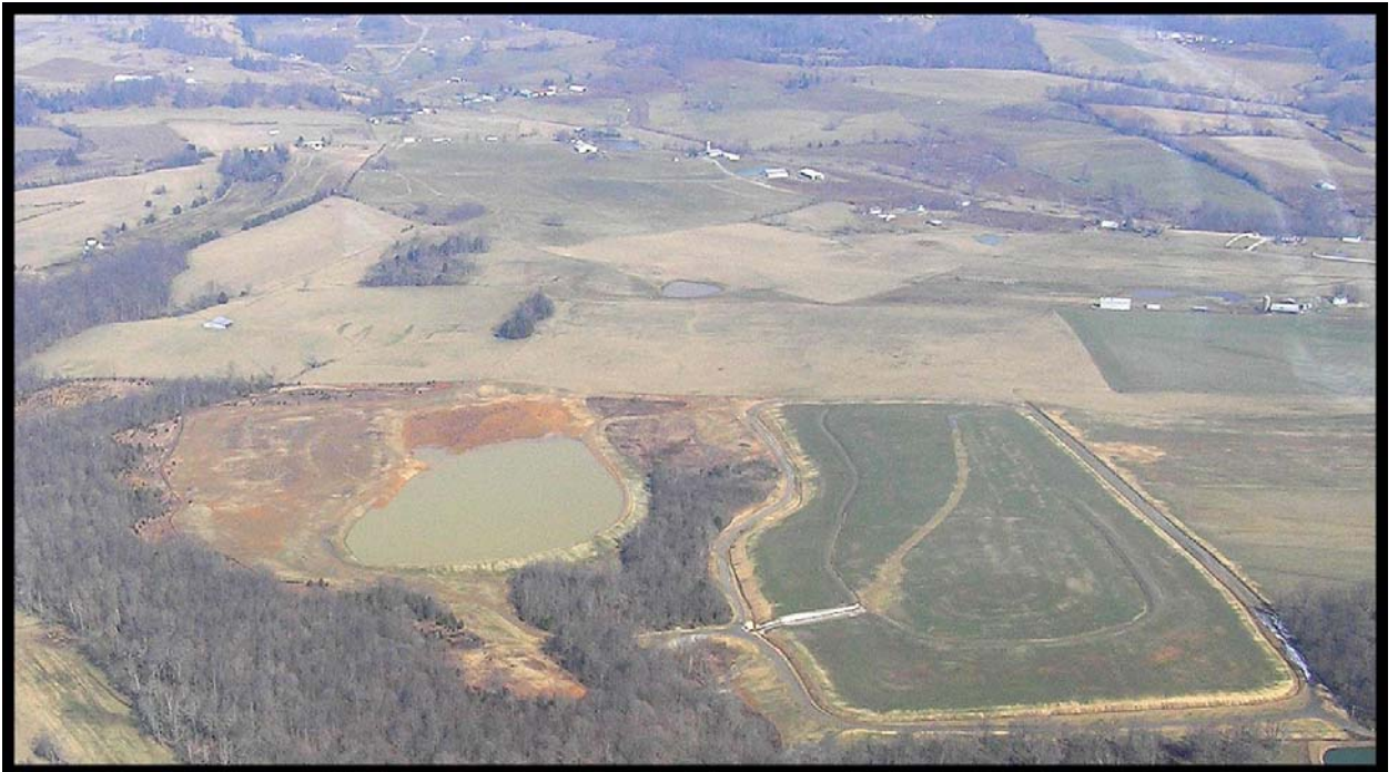
City of Campbellsville Landfill- Completed Closure Construction
