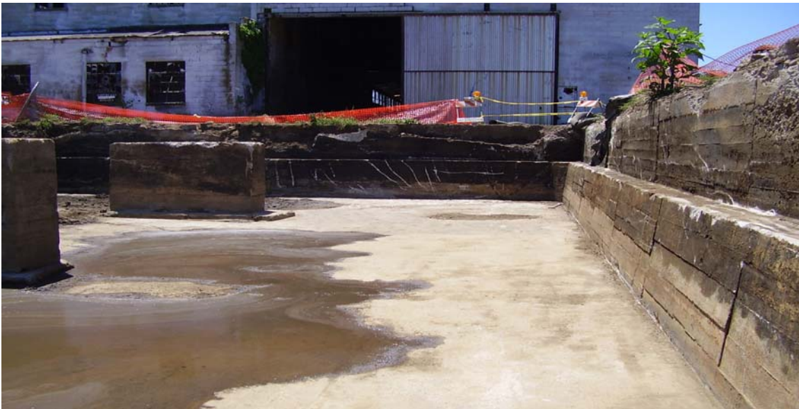
Derby Tank Car Project –prewater removal (after clean up)
