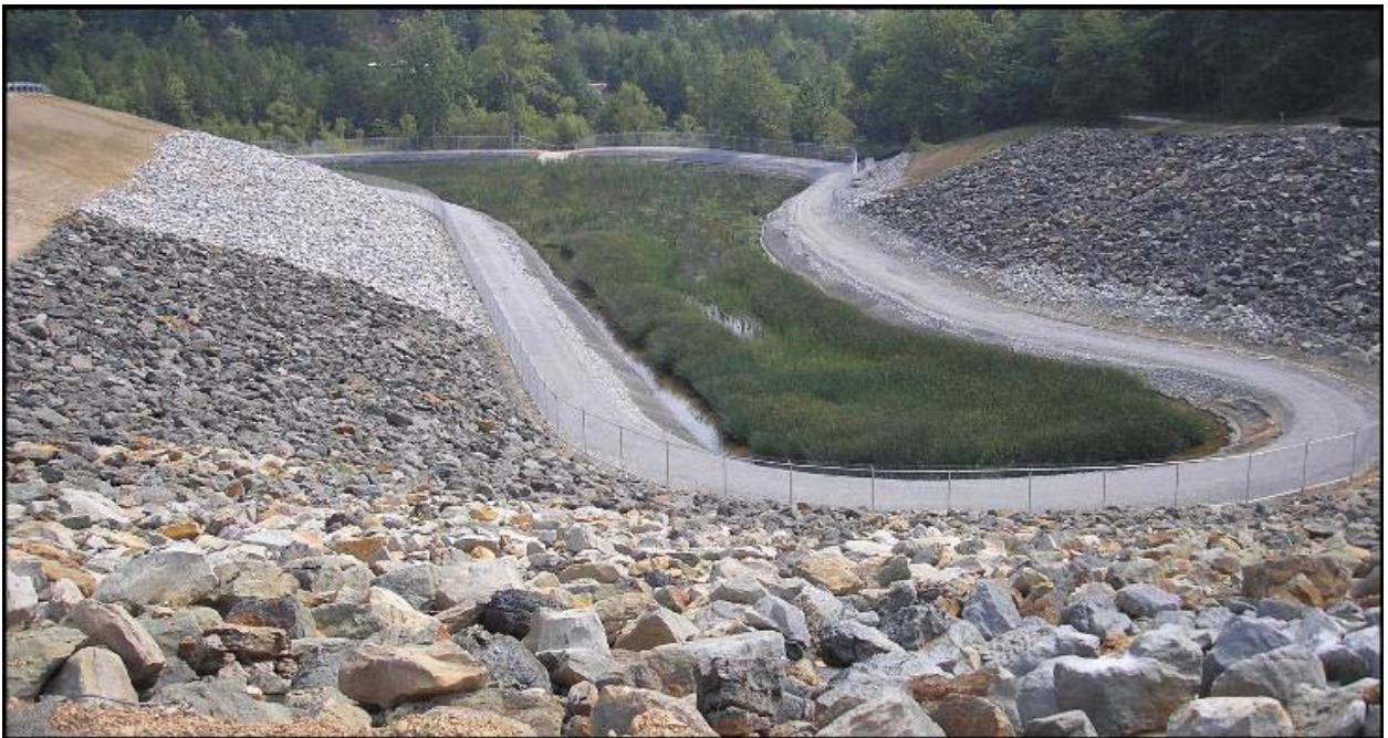
City of Manchester Landfill- Constructed Wetland Completed
