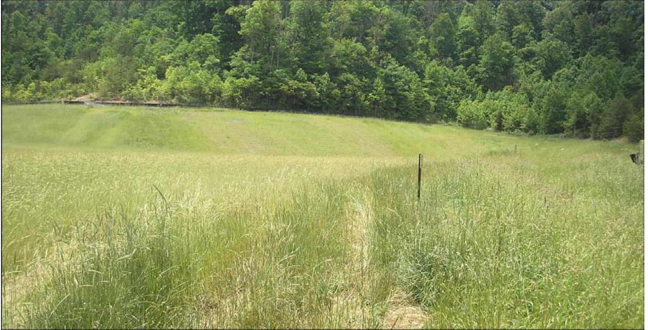
City of Manchester Landfill- Completed Final Cover Construction
