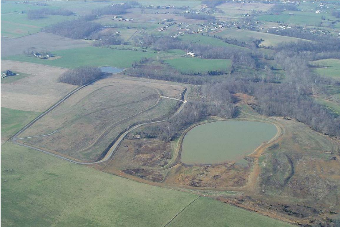
City of Campbellsville's solid waste landfill site post closure.
