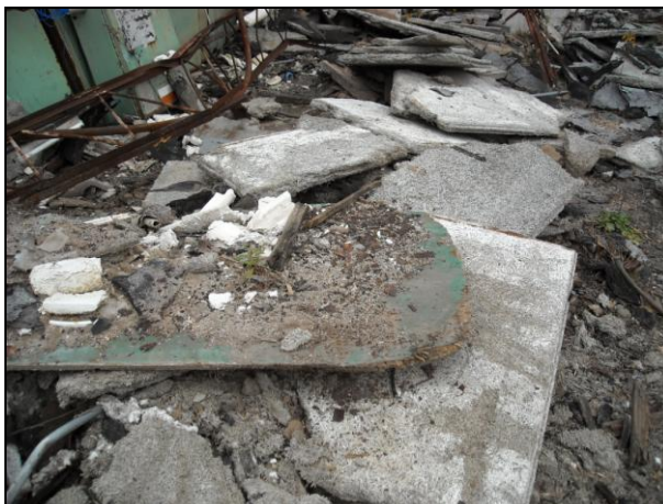
Asbestos containing tiles- photo taken November 2010
