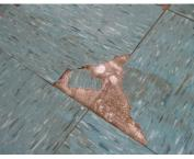
Example of non-friable asbestos floor tile. Photo: Townsville Asbestos Pty Ltd.
