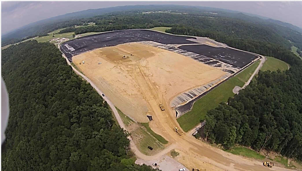
Aerial View of MFP Final Cap Construction Looking Northeast on June 30, 2015 Photo by Scott Wilburn
