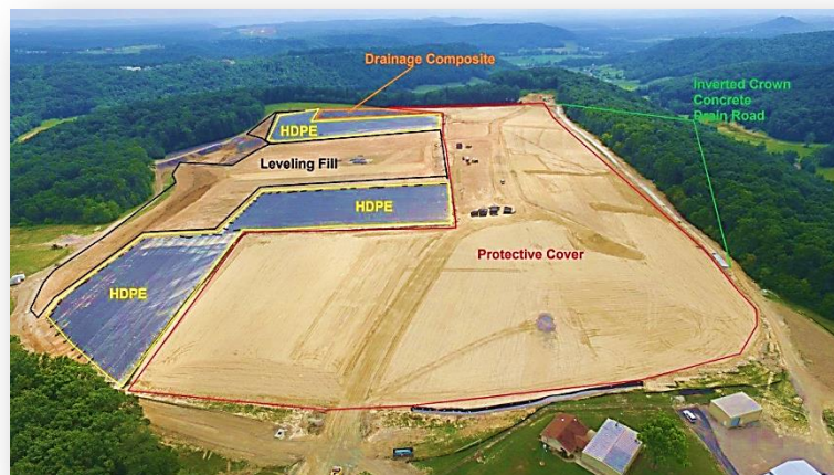
Aerial View of MFP Cap Construction Looking South in June 2016 Photo by Scott Wilburn
