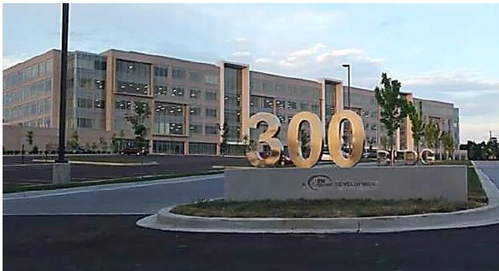
New State Office Building at 300 Sower Blvd., Frankfort, Kentucky EEC Photo
