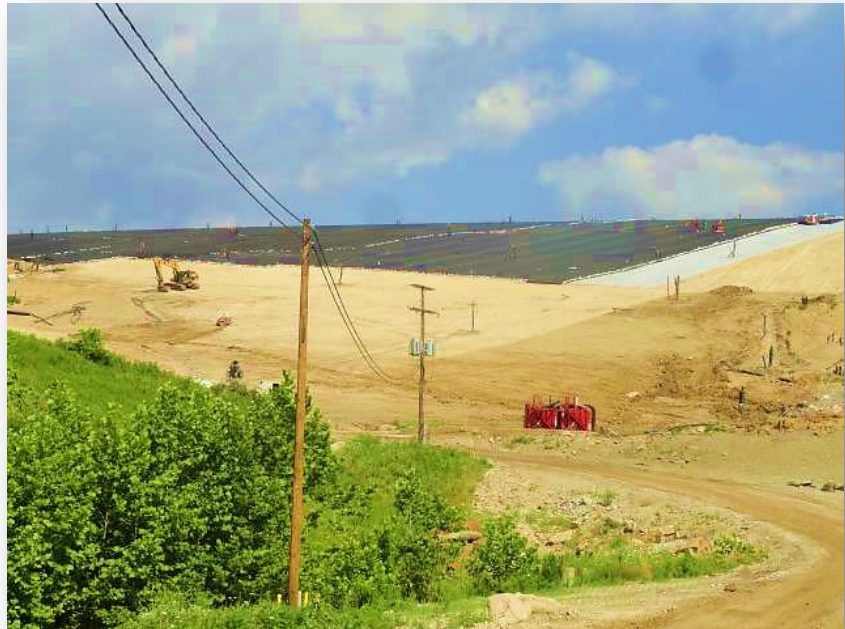
Big Run Landfill, Installation of Final Cap, South Slope, Units 1 & 2, Phase
