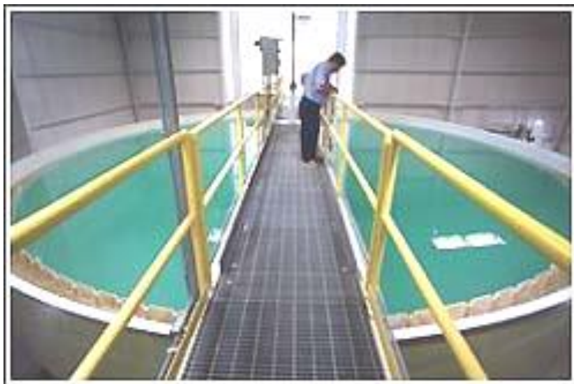
Top View of an Upflow Clarifier
