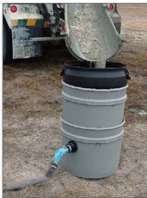
Figure 3. Concrete washout filter
