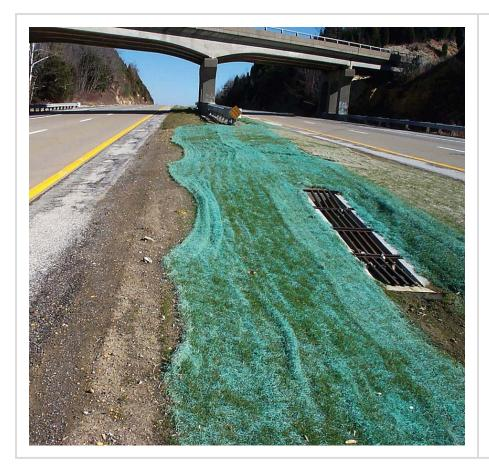
Good application of erosion control blanket to stabilize shoulder and protect storm drain, but too few staples used along the top edge.
