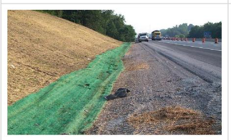
Very good installation of erosion control blanket in seeded ditch below wellmulched slope on highway project.
