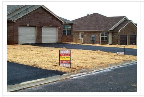
Excellent application of handscattered straw mulch in new residential subdivision. Work sites must be seeded and mulched as soon as final grade is established. Crimp mulch into soil with dozer tracking or disk harrows set straight to prevent straw from blowing.
