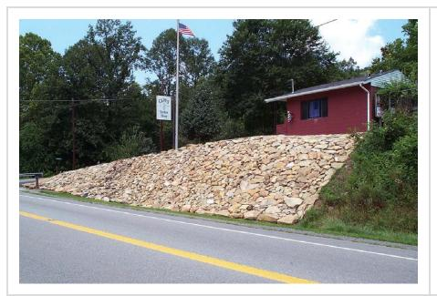
Good slope protection with permanent rock cover. This slope could have been protected with erosion control blankets or mats and seeded for a "softer" look.
