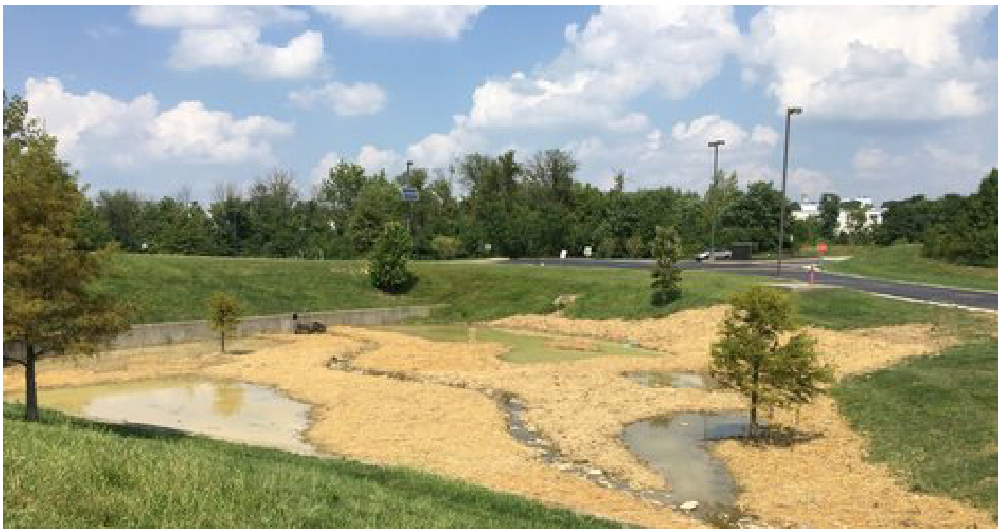
Figure 12. Stormwater project, Burlington, KY.
