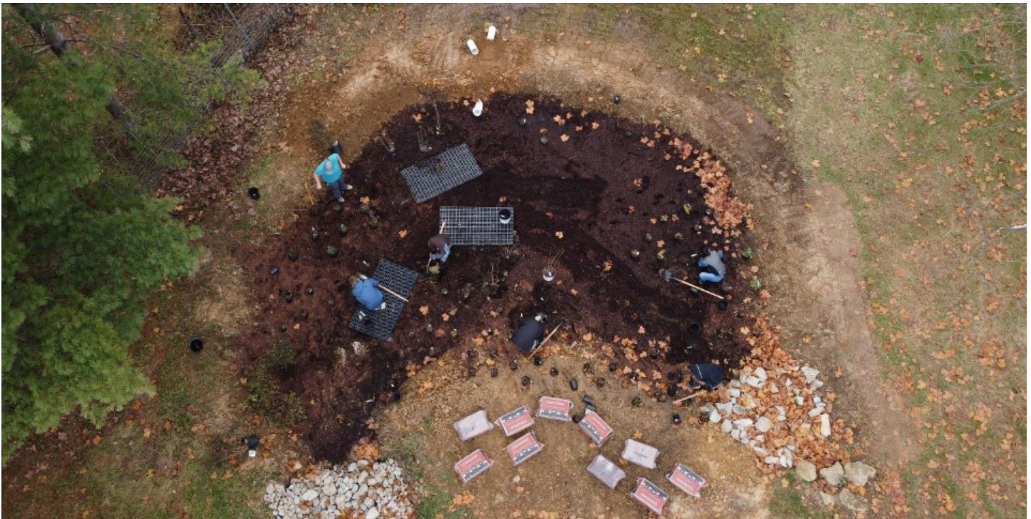
Figure 11. Rain garden construction at Yew Dell Gardens in Oldham County
