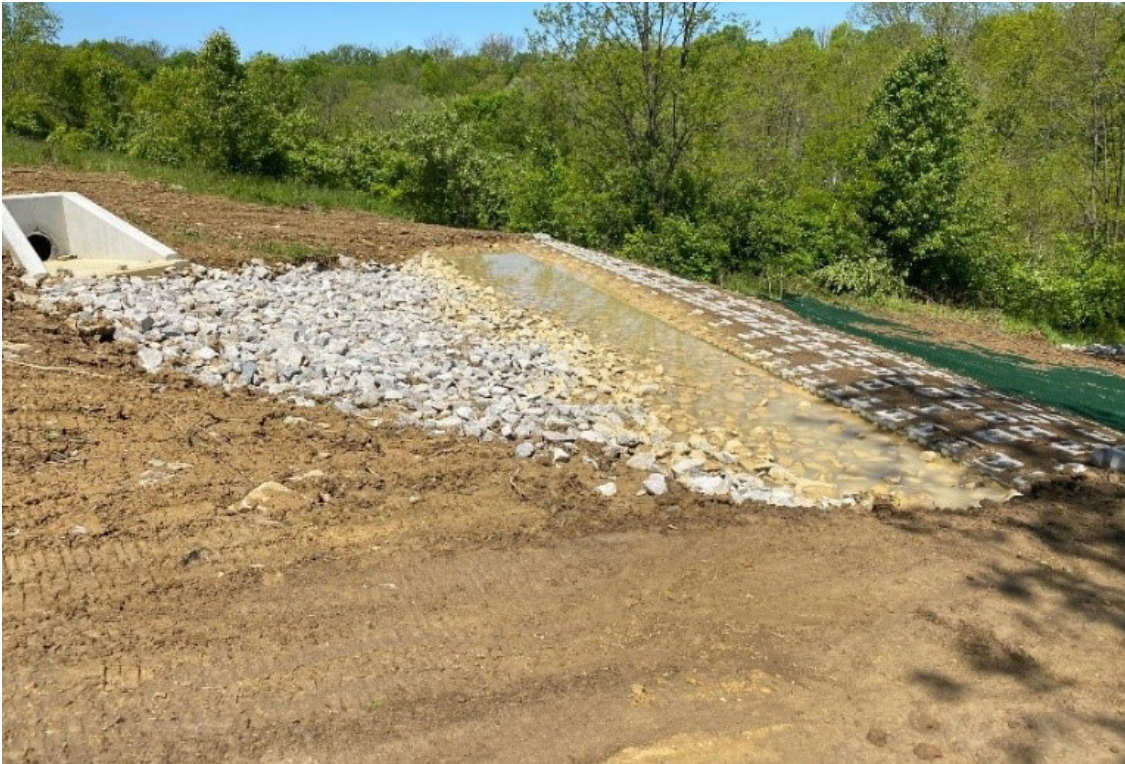
Figure 6. Level spreader best management practice
