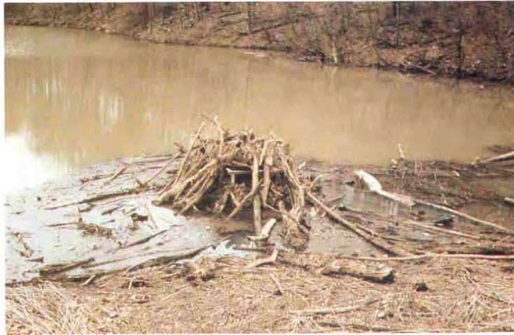
Photos Q and R: Collections of debris at the riser and shoreline: Debris had damaged trash rack on riser and further flows could reduce hydraulic capacities. Debris on shoreline should be removed as well as that on riser.
