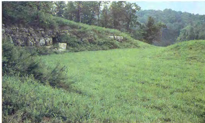
Photo D: A vegetated spillway. Grass is dense and mown just as on dam.
