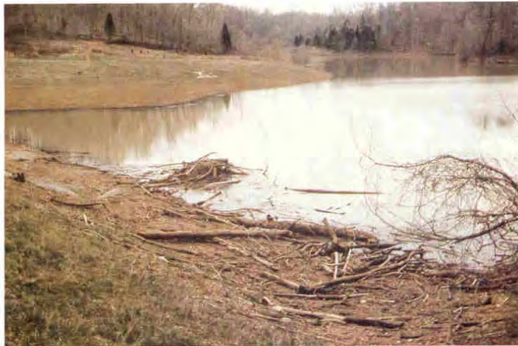
Photos Q and R: Collections of debris at the riser and shoreline: Debris had damaged trash rack on riser and further flows could reduce hydraulic capacities. Debris on shoreline should be removed as well as that on riser.
