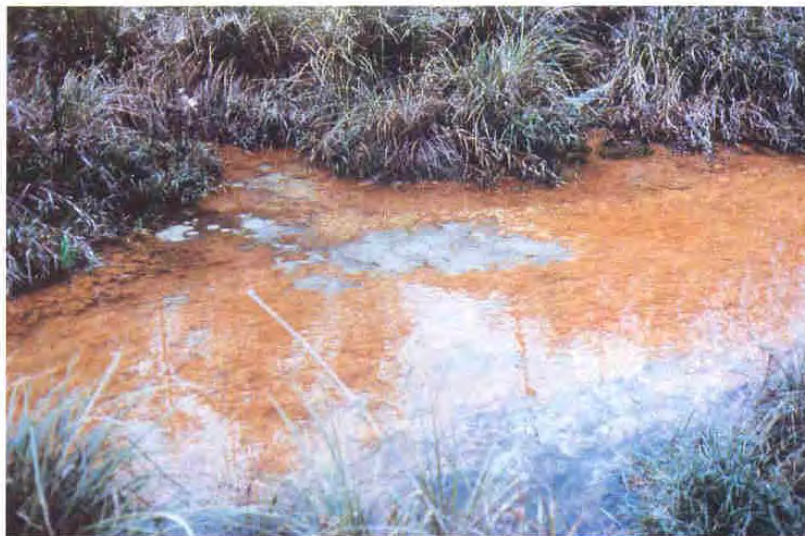
Photo F: Sand boils in an outlet channel below a dam. The seepage must be filtered and discharged.
