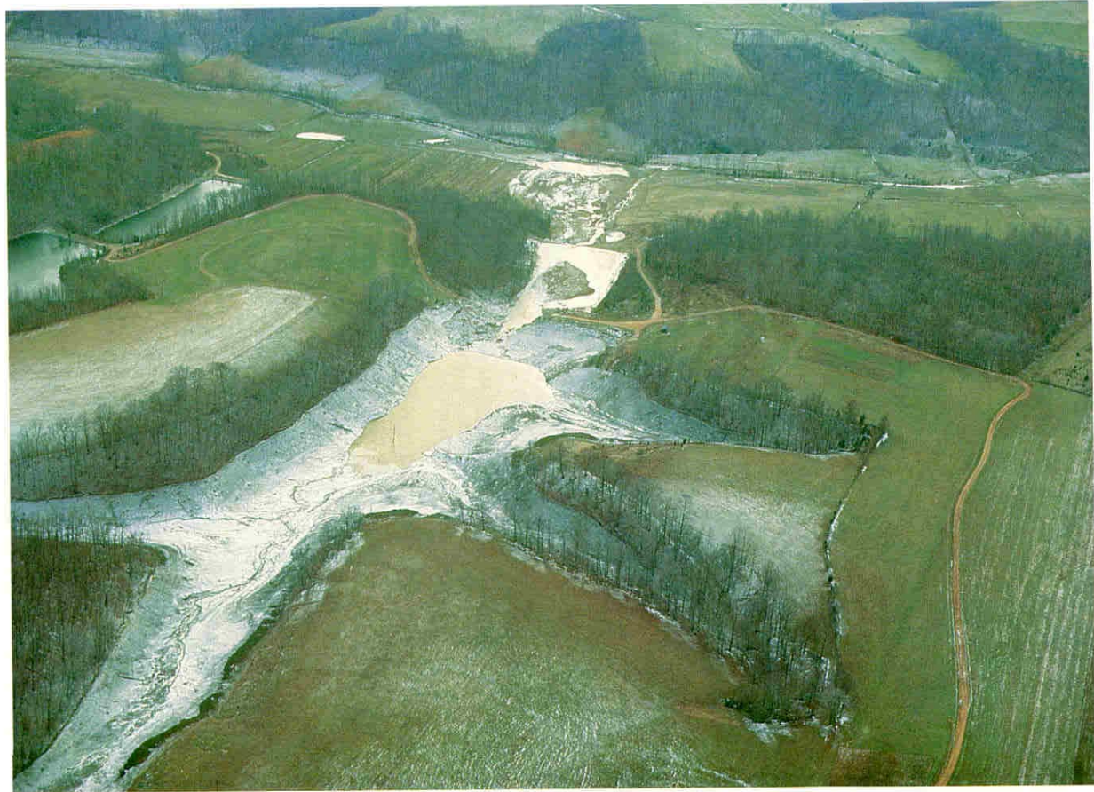
Caulk Dam Failure Taylor County, Kentucky December, 1973
