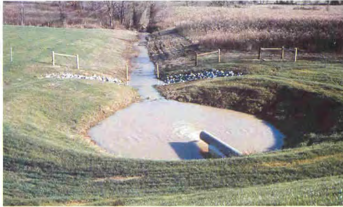
Photo C: An example of well maintained downstream slope and principal spillway.
