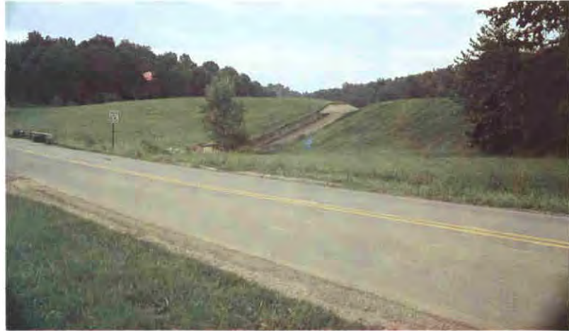
Photo A: An example of a well maintained dam and spillway.
