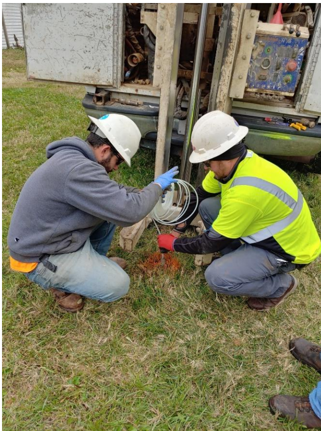
Photo 16: Drilling Company Installing the Soil Vapor Probes. Photo by Nathan Hancock.
