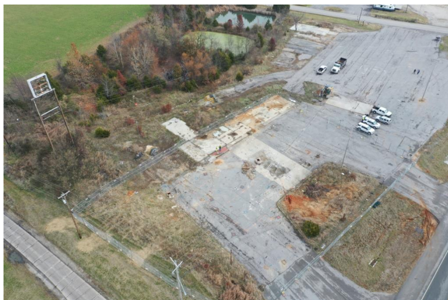
Photo 20: Drone photo of Sammy's Market UST site immediately prior to soil-mixing. Photo by Belle Thomas.
