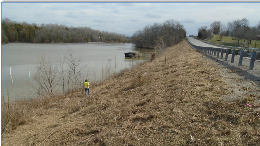
Upstream Slope and Reservoir of Willisburg Dam, February 2023
