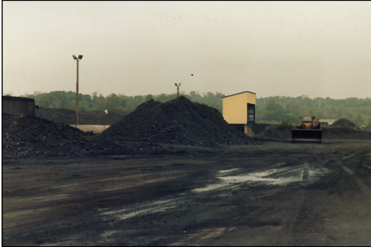
Owensboro Coal Dock circa 1985. Kentucky Energy and Environment Cabinet archives.
