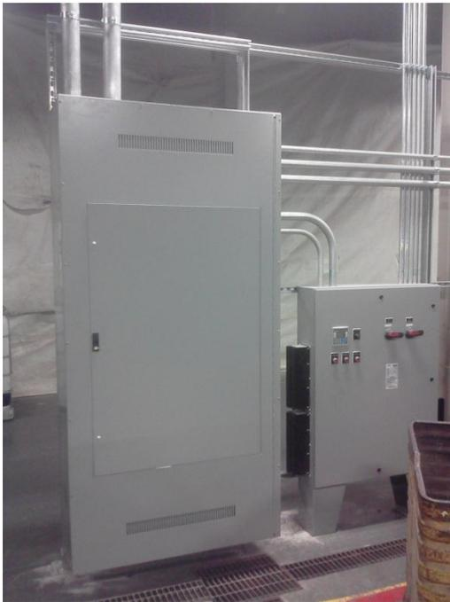
The picture above is of the electric panels that control a set of electric immersion heaters.
