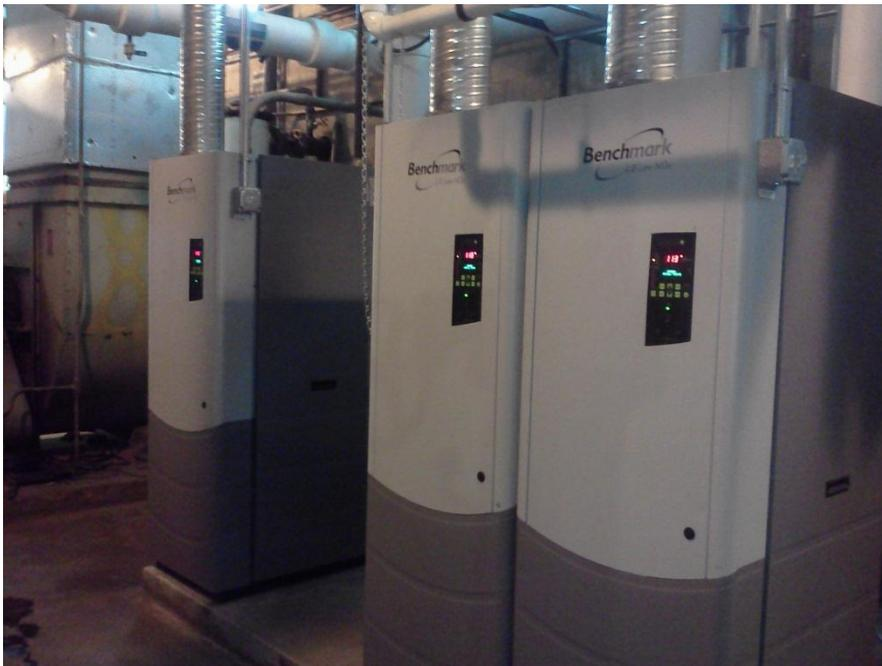
Above is a picture of the hot water boilers that supply heat to the front office areas.
