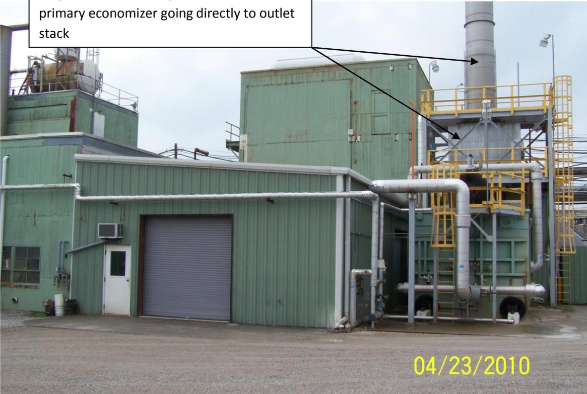
New Condensing Economizer with exhaust gas from two boilers being rerouted to take advantage of remaining "latent heat"
