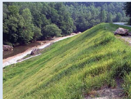
Rock Creek bank after restoration
