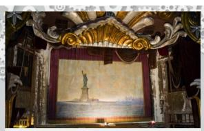
Before any asbestos remediation could take place at the Columbia Theatre, the fire curtain, which is made of asbestos, had to be restored and encapsulated. Afterward, the Columbia Club was able to use its grant from the CCF to remediate a majority of the other asbestos sources in the building.
