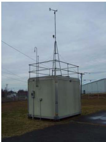
The monitoring site is a stationary equipment shelter located on the grounds of the DOT Garage on KY1008 in Franklin, Kentucky. The sample inlet is 61 meters from the nearest road. The most recent site inspection was conducted on December 17, 2009. Upon inspection, the sample line and monitor were found to be in good condition. The site meets the requirements of 40 CFR 58, Appendices C, D, E and G.
