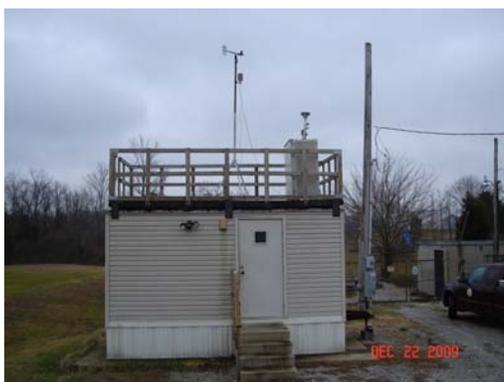
The monitoring site is a stationary equipment shelter located on the grounds of the Bates Elementary School in Louisville, Kentucky. The sample inlets are 4.0 meters above ground level and 305 meters from the nearest road. The most recent site inspection was conducted on December 21, 2009. The air monitoring site was found to be in accordance with 40 CFR Part 58, Appendices C, D, E and G.
