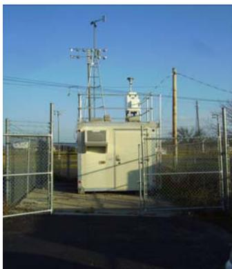
The monitoring site is a stationary equipment shelter located in a fenced-in area near the intersection of Second and Carpenter Streets in Shepherdsville, Kentucky. The sample inlets are 56 meters from the nearest road. The most recent site inspection was conducted on November 20, 2009. Upon inspection, the sample lines and monitors were found to be in good condition. The site meets the requirements of 40 CFR 58, Appendices C, D, E and G.
