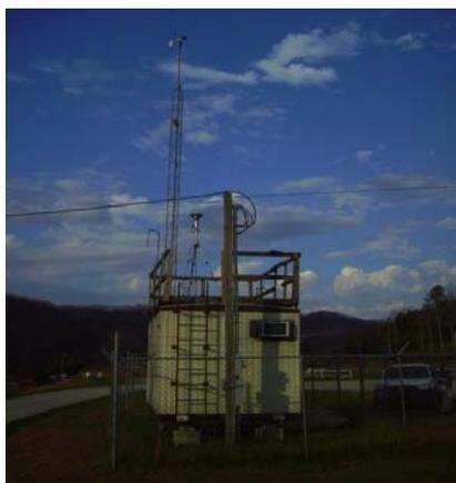
The monitoring site is a stationary equipment shelter located on the grounds of the Perry County Horse Park in Hazard, Kentucky. The sample inlets 33 meters from the nearest road. The most recent site inspection was conducted on November 17, 2009. Upon inspection the sample lines and monitors were found to be in good condition. This site meets the requirements of 40 CFR 58, Appendices C, D, E and G.
