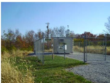
The monitoring site is a stationary equipment shelter located on farmland owned by the Northern Kentucky University in Highland Heights, Kentucky. The sample inlets are 22 meters from the nearest road, which is a dirt service drive for a radio tower. The most recent site inspection was conducted on November 4, 2009. Upon inspection, the sample lines and monitors were found to be in good condition. The site meets the requirements of 40 CFR 58, Appendices C, D, E and G.
