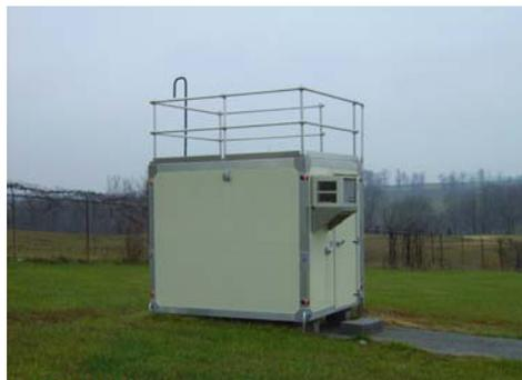
The monitoring site is a stationary equipment shelter located on the grounds of the Kentucky DOT Highway Garage in Buckner, Kentucky. The sample inlet is 76 meters from the nearest road. The most recent site inspection was conducted on December 18, 2009. Upon inspection, the sample line and monitor were found to be in good condition. The site meets the requirements of 40 CFR 58, Appendices C, D, E and G.
