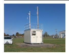
The monitoring site is a stationary equipment shelter located on the grounds of the Kentucky Transportation Cabinet garage in Nicholasville, Kentucky. The sample inlets are 110 meters from the nearest road. Upon inspection, the sample inlets and monitors were found to be in good condition. The site meets the requirements of 40 CFR 58, Appendices C, D, E and G.
