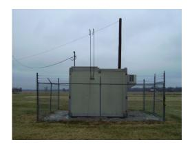
The monitoring site is a stationary equipment shelter located on the grounds of the former Lewisport Elementary School in Lewisport, Kentucky. The sample inlet is 57 meters from the nearest road. Upon inspection, the sample line and monitor were found to be in good condition. The site meets the requirements of 40 CFR 58, Appendices C, D, E and G.
