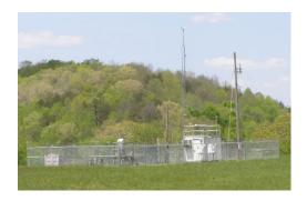
The monitoring site is a stationary equipment shelter in a fenced area located in a remote section of Camp Webb in Grayson, Kentucky. The nearest road is a service road to the site and is 98 meters from the site. Upon inspection, the sample lines and monitors were found to be in good condition. The site meets the requirements of 40 CFR 58, Appendices A, C, D, and E.
