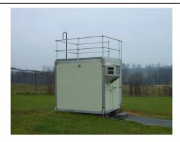
The monitoring site is a stationary equipment shelter located on the grounds of the Kentucky DOT Highway Garage in Buckner, Kentucky. The sample inlet is 51 meters from the nearest road. Upon inspection, the sample line and monitor were found to be in good condition. The site meets the requirements of 40 CFR 58, Appendices C, D, E and G.
