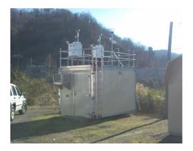
The monitoring site is a stationary equipment shelter located behind the KYTC District Office building in Pikeville, KY. The sample inlets are 91.1 meters from the nearest road. Upon inspection the sample lines and monitors were found to be in good condition. This site meets the requirements of 40 CFR 58, Appendices A, C, D, E and G.
