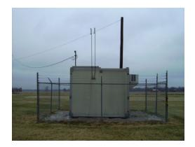
The monitoring site is a stationary equipment shelter located on the athletic fields of the former Lewisport Consolidated Elementary School in Lewisport, Kentucky. The sample inlet is 55.3 meters from the nearest road. Upon inspection, the sample line and monitor were found to be in good condition. The site meets the requirements of 40 CFR 58, Appendices A, C, D, and E.
