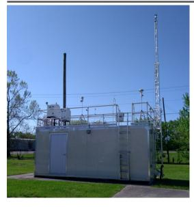
The monitoring site is a stationary equipment shelter located on the grounds of the Firearms Training Center in Louisville, Kentucky. The sample inlet is 4.5 meters above ground level and 53.5 meters from the nearest road. Upon inspection, the sample lines and monitors were found to be in good condition. The air monitoring site meets the criteria established by 40 CFR Part 58, Appendices C, D, E and G.
