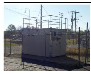
The monitoring site is a stationary equipment shelter located in a fenced-in area near the intersection of Second and Carpenter Streets in Shepherdsville, Kentucky. The sample inlets are 66.4 meters from the nearest road. Upon inspection, the sample lines and monitors were found to be in good condition. The site meets the requirements of 40 CFR 58, Appendices A, C, D, and E.
