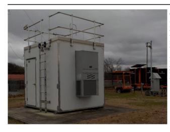
The monitoring site is a stationary equipment shelter located on the grounds of the Livingston County Road Dept. facility in Smithland, Kentucky. The sample inlets are 138.7 meters from the nearest road. Upon inspection, the sample lines and monitors were found to be in good condition. The site meets the requirements of 40 CFR 58, Appendices A, C, D, and E
