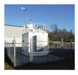
The monitoring site is a stationary equipment shelter located on the grounds of the Middlesboro Airport in Middlesboro, Kentucky. The sample inlets are 94.2 meters from the nearest road. Upon inspection the sample lines and monitors were found to be in good condition. The site meets the requirements of 40 CFR 58, Appendices A, C, D, and E.
