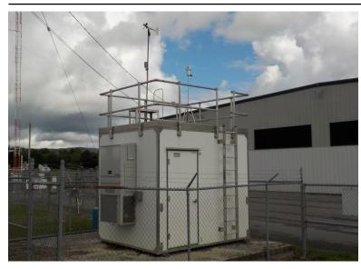
The monitoring site is a stationary equipment shelter located on the grounds of the Middlesboro Airport in Middlesboro, Kentucky. The sample inlets are 94.2 meters from the nearest road. Upon inspection the sample lines and monitors were found to be in good condition. The site meets the requirements of 40 CFR 58, Appendices A, C, D, and E.
