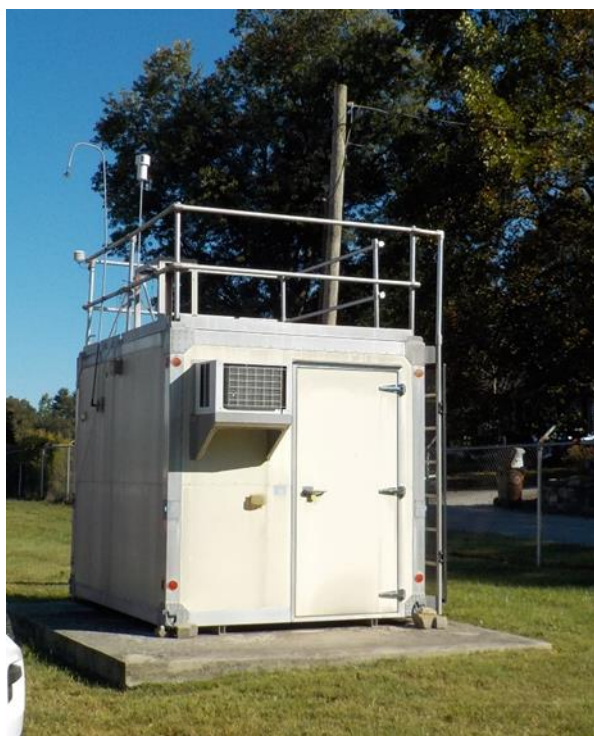
Figure 1: Picture of the Somerset air monitoring station.
