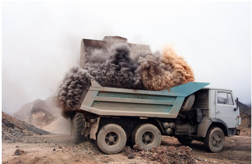
Fugitive emissions from land clearing for construction. State regulation requires control measures to reduce fugitive emissions and their impact on air quality. (Photo: Shutterstock)
