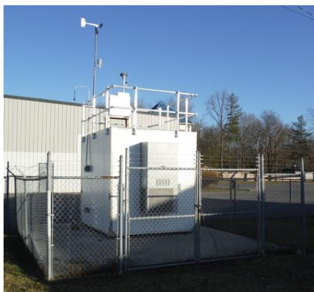
The monitoring site is a stationary equipment shelter located on the grounds of the Middlesboro Airport in Middlesboro, Kentucky. The sample inlets are 93.5 meters from the nearest road. Upon inspection the sample lines and monitors were found to be in good condition. The site meets the requirements of 40 CFR 58, Appendices A, C, D, and E.
