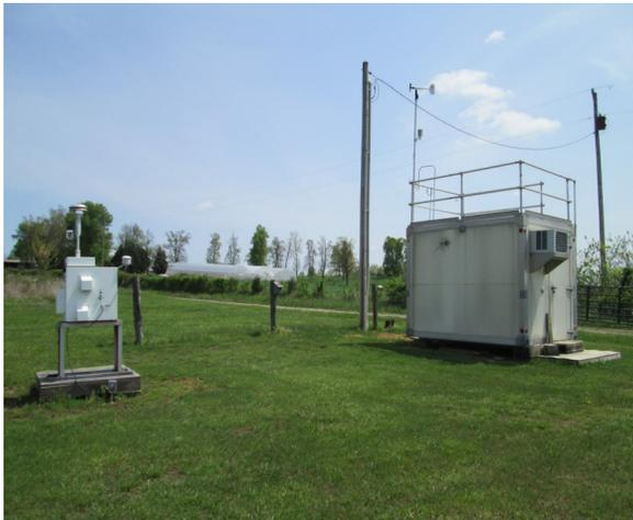
The monitoring site consists of a PM<sub>2.5</sub> monitoring platform and an adjacent stationary equipment shelter. The site is located in a field on the property of a private residence, located at 10800 Pilot Rock Road in Hopkinsville, Kentucky. The sample inlets are 116 meters from the nearest road. Upon inspection, the sample inlets and monitors were found to be in good condition. The site meets the requirements of 40 CFR 58, Appendices A, C, D and E.
