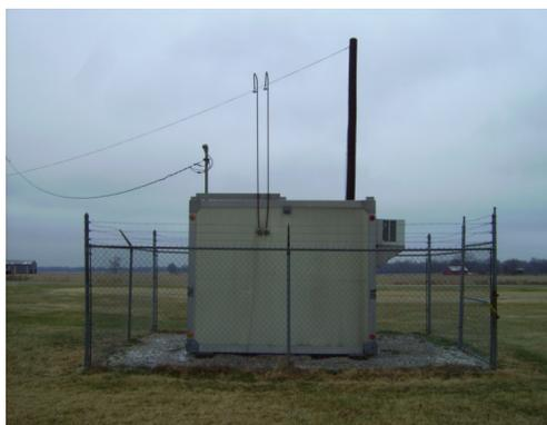
The monitoring site is a stationary equipment shelter located on the athletic fields of the former Lewisport Consolidated Elementary School in Lewisport, Kentucky. The sample inlet is 55.3 meters from the nearest road. Upon inspection, the sample line and monitor were found to be in good condition. The site meets the requirements of 40 CFR 58, Appendices A, C, D, and E.
