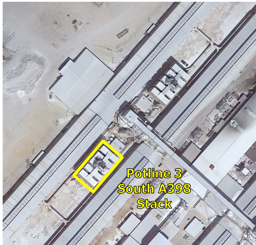
Figure 2-8. Aerial Image of Potline 3 South A-398 Stack Configuration
