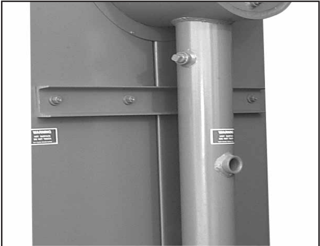
Figure 3-3: Feed Water Inlet Steam Boiler
