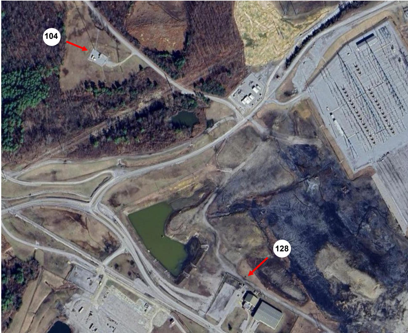
104 - Cell Phone Tower (Two-Way Radio) Emergency Diesel Engine 128 - Emergency Telecommunications Propane Generator
