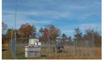
The monitoring site is a stationary equipment shelter in a fenced area located in a remote section of Camp Webb in Grayson, Kentucky. The nearest road is a service road to the site and is 106 meters from the site. Upon inspection, the sample lines and monitors were found to be in good condition. The site meets the requirements of 40 CFR 58, Appendices A, C, D, E, and G.
