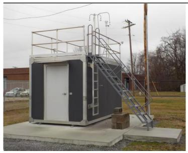
The monitoring site is a stationary equipment shelter located on the grounds of Paducah Area Transit System in Paducah, Kentucky. The sample inlets are 30 meters from the nearest road. The site meets the requirements established by 40 CFR 58, Appendices A, C, D, E, and G. This site was formally Jackson Purchase (21-145-1024). The property owners were expanding operations and the site had to be relocated as quickly as possible. Paducah Transit is 2.8 miles NW of the Jackson Purchase site.
