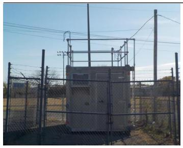
The monitoring site is a stationary equipment shelter located in a fenced-in area near the intersection of Second and Carpenter Streets in Shepherdsville, Kentucky. The sample inlets are 58 meters from the nearest road. Upon inspection, the sample lines and monitors were found to be in good condition. The site meets the requirements of 40 CFR 58, Appendices A, C, D, E, and G.
