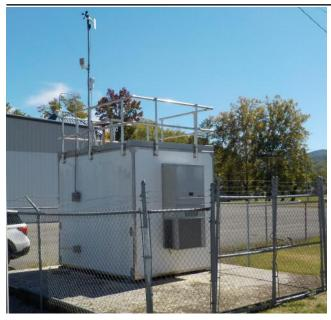
The monitoring site is a stationary equipment shelter located on the grounds of the Middlesboro Airport in Middlesboro, Kentucky. The sample inlets are 96 meters from the nearest road. Upon inspection the sample lines and monitors were found to be in good condition. The site meets the requirements of 40 CFR 58, Appendices A, C, D, E and G.
