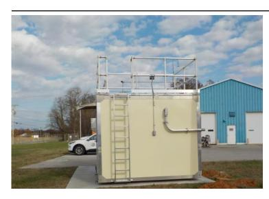
The monitoring site is a stationary equipment shelter located on the grounds of the KYTC Garage on Harding Road (KY1008) in Franklin, Kentucky. The sample inlet is 42.5 meters from the nearest road. Upon inspection, the sample line and monitor were found to be in good condition. The site meets the requirements of 40 CFR 58, Appendices A, C, D, and E.
