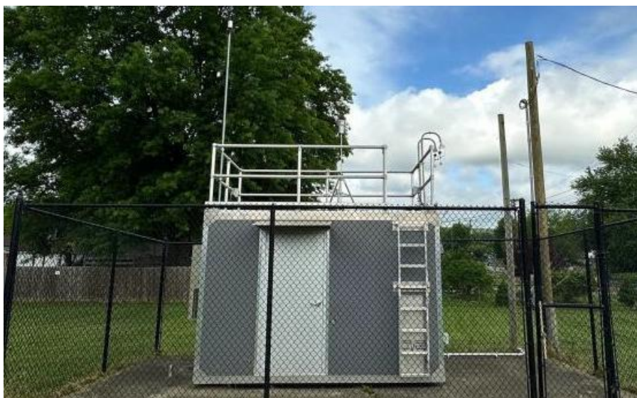
Figure 45: Watson Lane Air Monitoring Shelter
