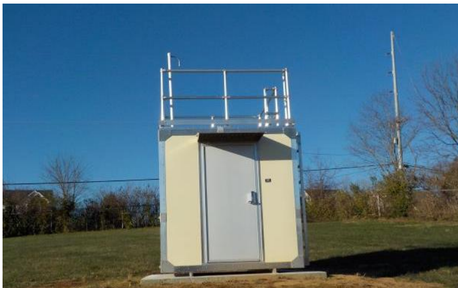
Figure 43: Buckner Air Monitoring Shelter
