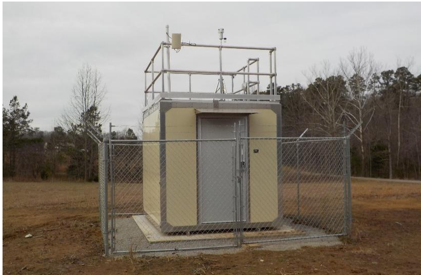
Figure 15: Pennyrile Forest Air Monitoring Shelter
