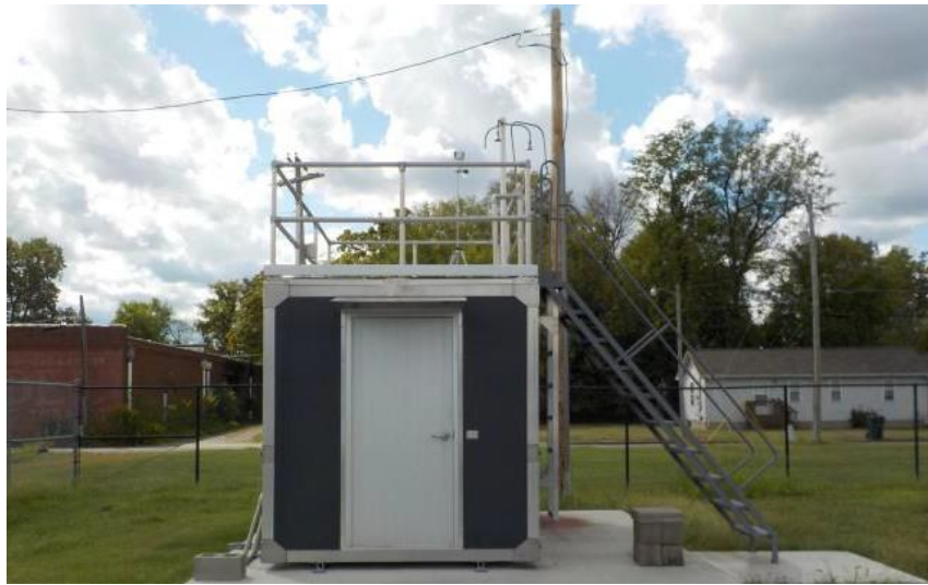
Figure 65: Paducah Transit Air Monitoring Shelter
