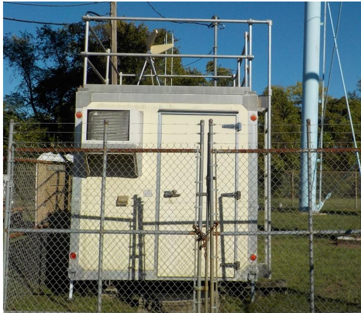
Figure 31: Worthington Air Monitoring Shelter
