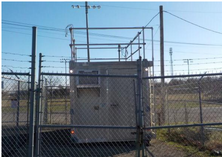
Figure 41: Shepherdsville Air Monitoring Shelter
