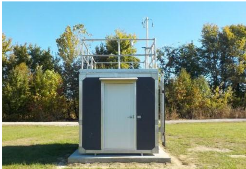
Figure 59: Meadow Lands Air Monitoring Shelter
