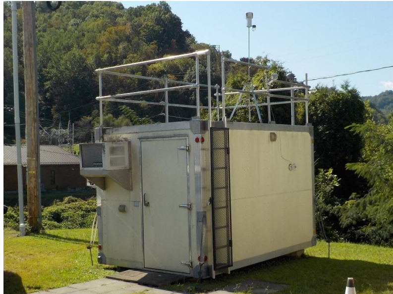
Figure 75: Pikeville Primary Air Monitoring Shelter
