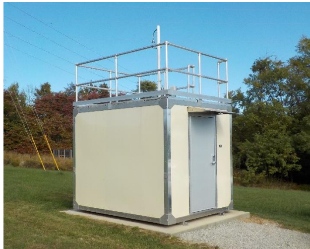
Figure 9: Nature Center Air Monitoring Shelter
