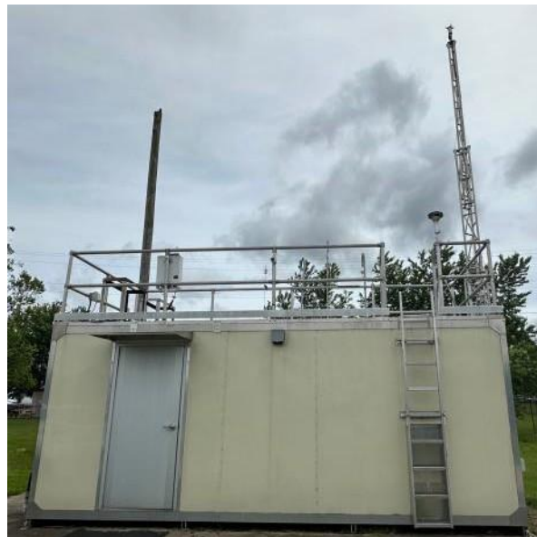
Figure 56: Algonquin Parkway Air Monitoring Shelter
