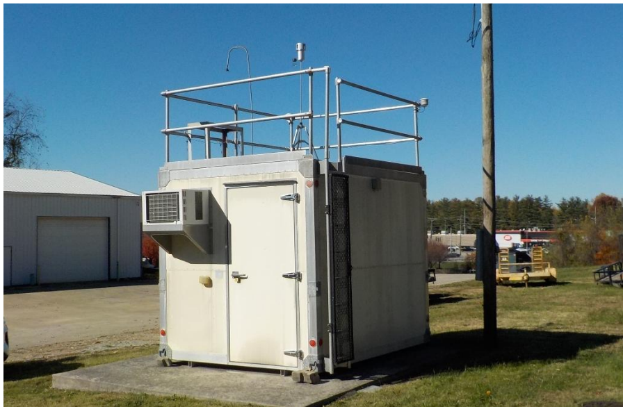
Figure 78: Somerset Air Monitoring Shelter
