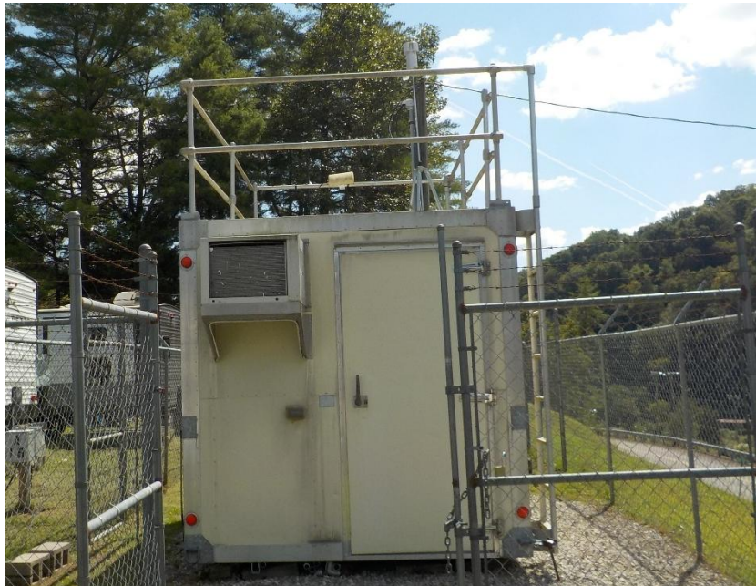
Figure 86: Hazard Air Monitoring Shelter
