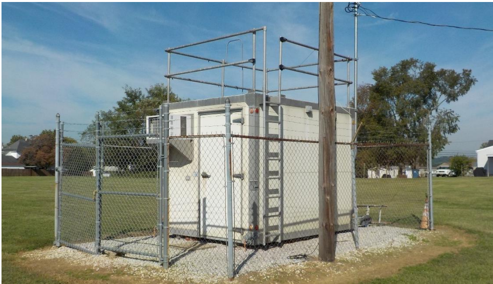
Figure 84: Lewisport Air Monitoring Shelter
