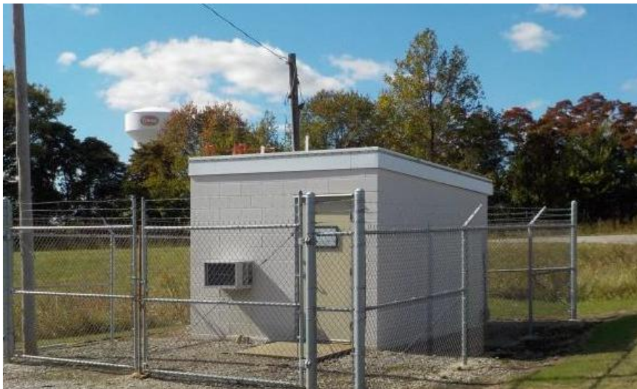
Figure 71: Sebree Air Monitoring Shelter
