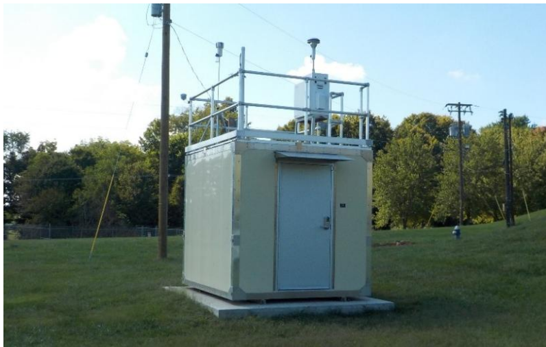
Figure 18: Freeman Lake Air Monitoring Shelter
