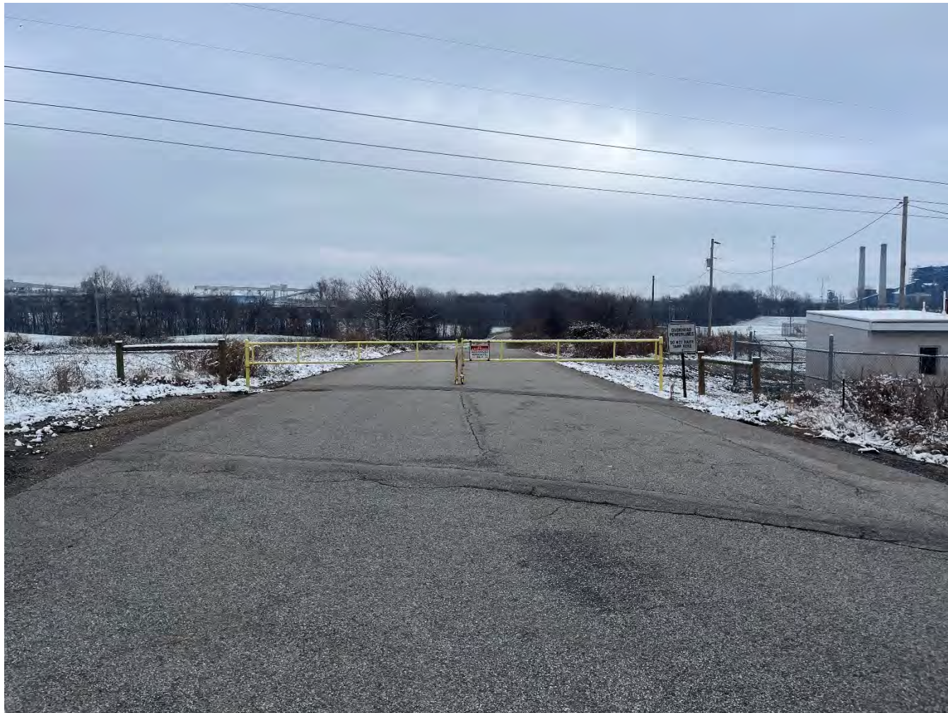
Figure 3 Rolling Gate at the Old Coal Truck Access Road Entrance
