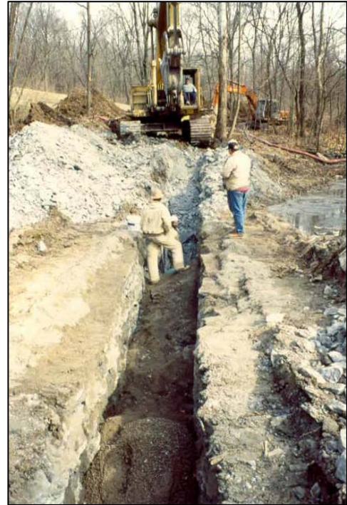
Trenching across or along a stream channel requires a US ACE permit and a KDOW water quality certification.
