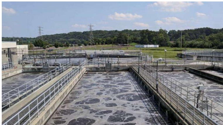
Figure 10.6 Activated Sludge Facility
