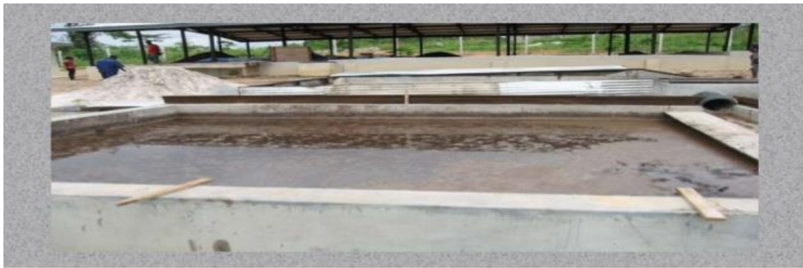
Figure 18.7 Sand Drying Bed Examples
