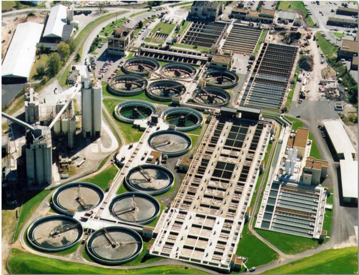
Figure 10.1 The Central Wastewater Treatment Plant, Nashville, Tennessee
