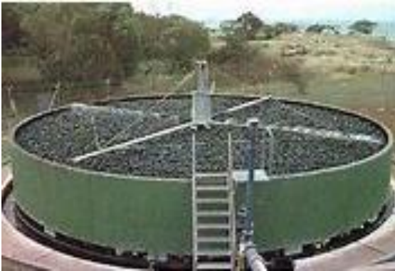
Figure 10.4 Trickling Filter
