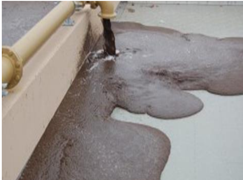
Figure 18.12 Loading Slurry onto Wedge-wire Bed
