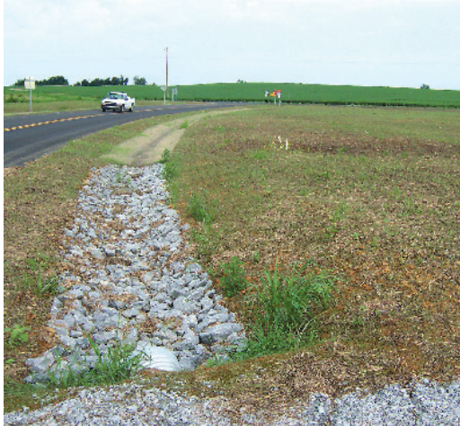
Here is a good example of rock-lined ditch. The seeding is a bit too thick on the side slopes.
