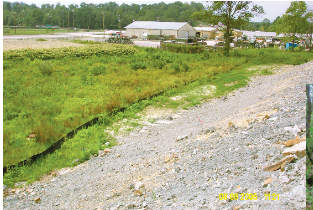
These are good examples of vegetated filter strips along a small swale (left) and large stream (below). Protect these areas during construction with flagging ribbon or signs.
