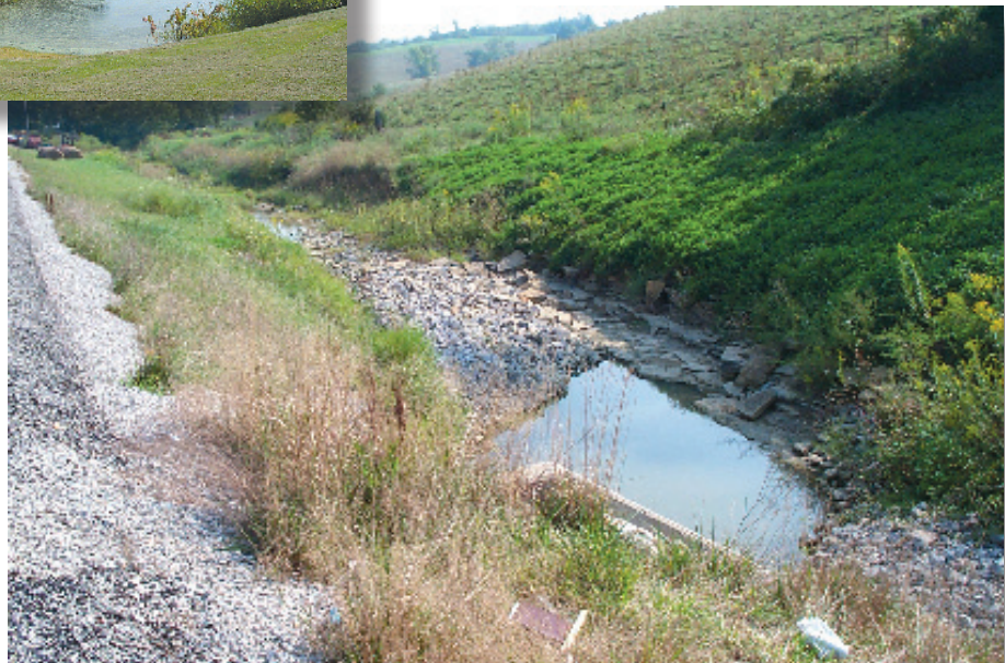
Filter strips along lakes and ponds (left) can include mowed access areas for fishing and other activities. Where severe scour forces are present, protect planted filter strips with turf reinforcement mats or other armoring to prevent bank erosion (below).
