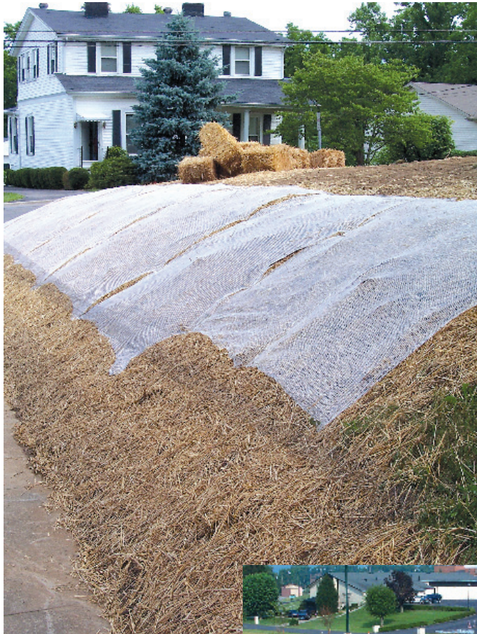
Use netting to secure loose straw on steep or long slopes. Above: Good coverage with straw mulch. Mulch alone can reduce erosion by more than 90 percent. Apply temporary or permanent mulch as soon as final grade is established.
