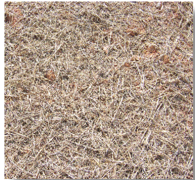
Visually inspect mulched areas to ensure uniform, sufficient coverage. Application must cover all bare areas, with less than 5 percent soil showing through mulch cover.
