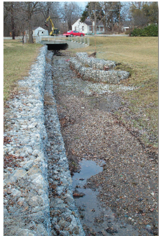
Gabions can protect banks in areas of high velocity flows. Some designers prefer TRMs in these situations, if space is available to slope banks back appropriately.
