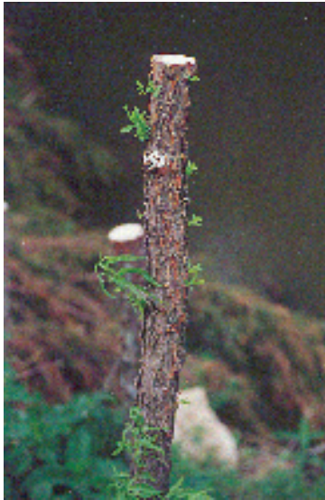
This is a sprouting willow stake. To avoid upside-down installation of stakes, require that the lower ends be cut at an angle, with the upper end cut flat, i.e., perpendicular to stake length.
