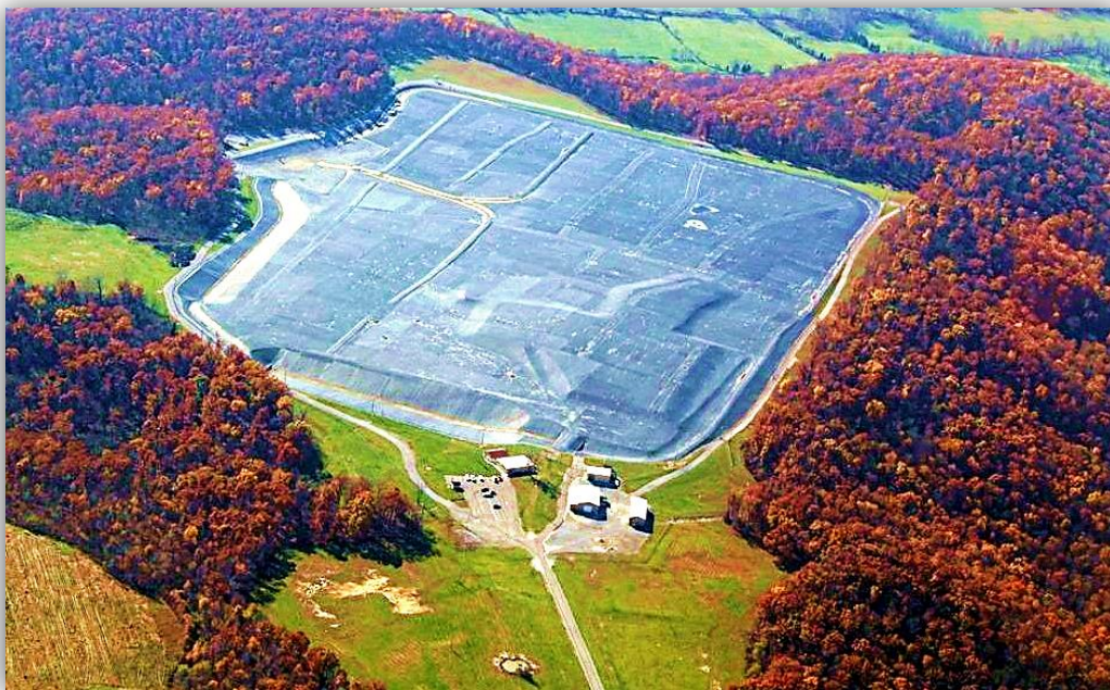
Aerial View of MFP before final closure activities - photo by Thomas Stewart, MFP
