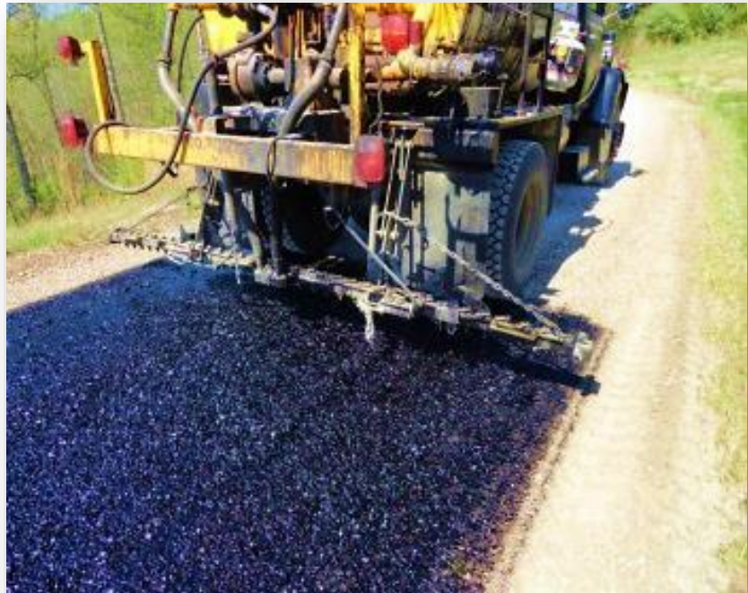
Application of Conventional-Asphalt Chip Seal in Whitley County, 2016 Photo by Christopher "Kitt" Tuttle
