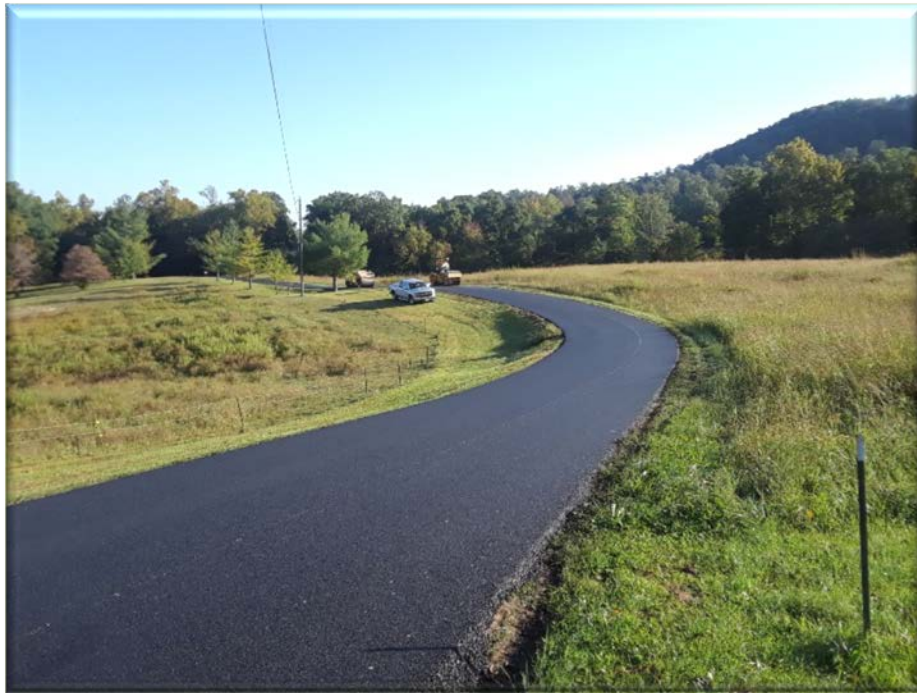
Photo 6: Rubber modified asphalt paving, Marion County. Photo by B.J. Bland
