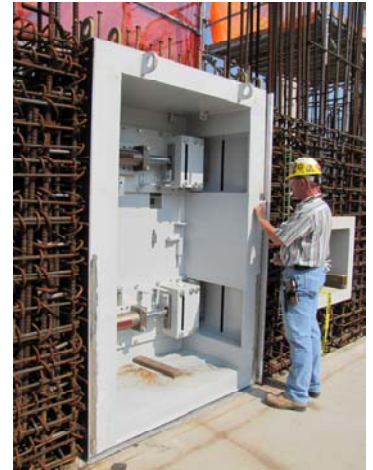
Dense rebar surrounds a thick steel door at the MDB
