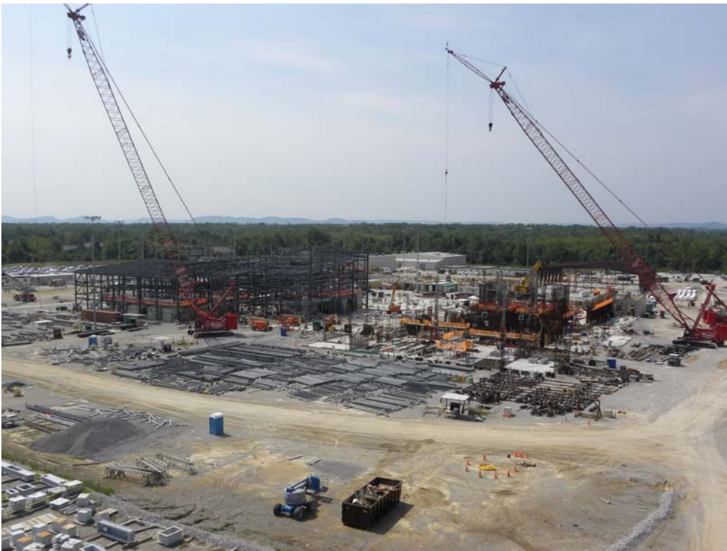
Aerial photo of the BGCAPP site, July 2010
