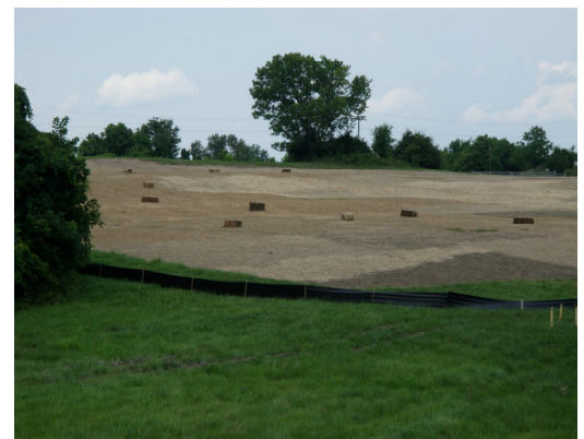
Hay applied to former lagoon area to encourage grass growth.
