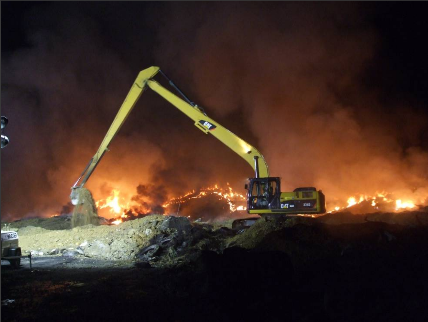
The cabinet contractor PECCO, Inc. places cover soil on the waste tires (EEC photo).
